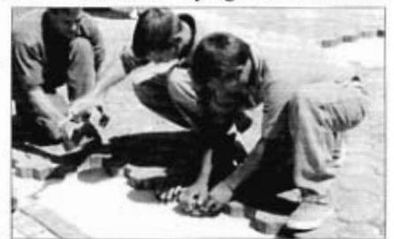
Three senior guys work on the patio.
